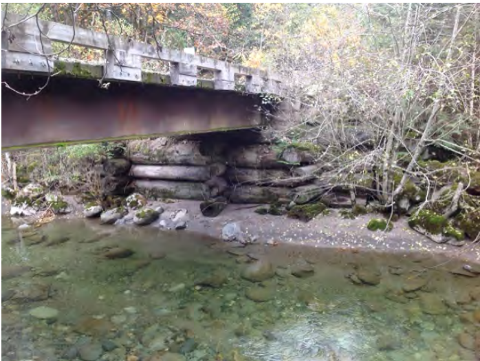
Right Bank Abutment when facing downstream
