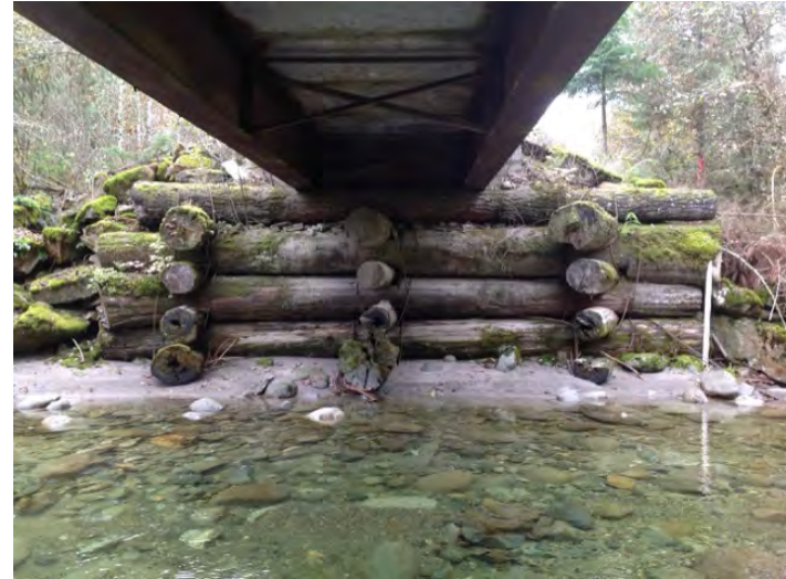
Left Bank Abutment when facing downstream
